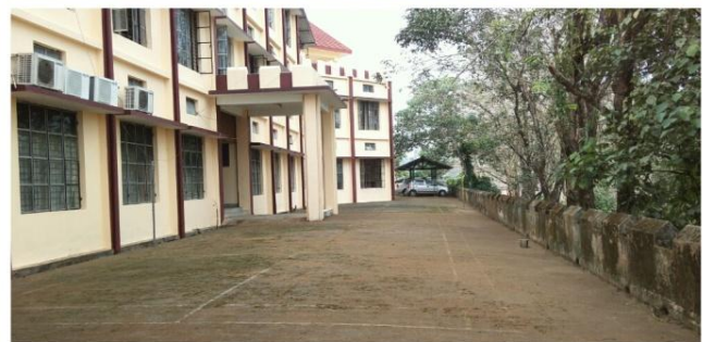
The backyard of Mechanical Engineering Department before and after cleaning
