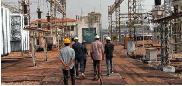
Industrial Visit to 220kV Switching station, KSEB substation, Pallom
